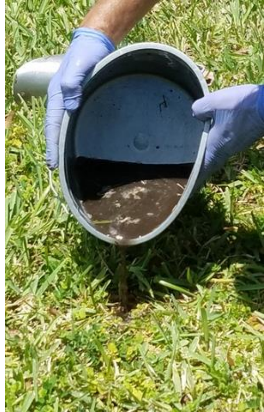
Figure 19. Pouring the slurry into the hole
